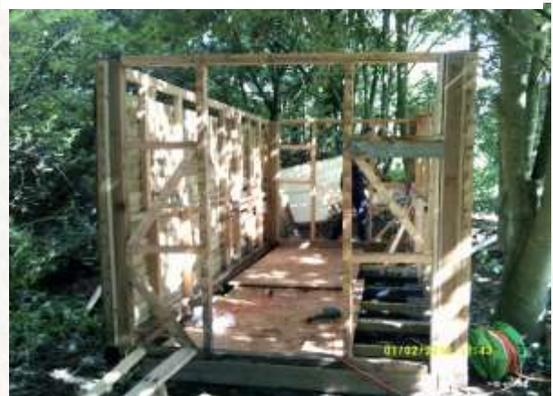
Figure 11. Wall frameworks complete
