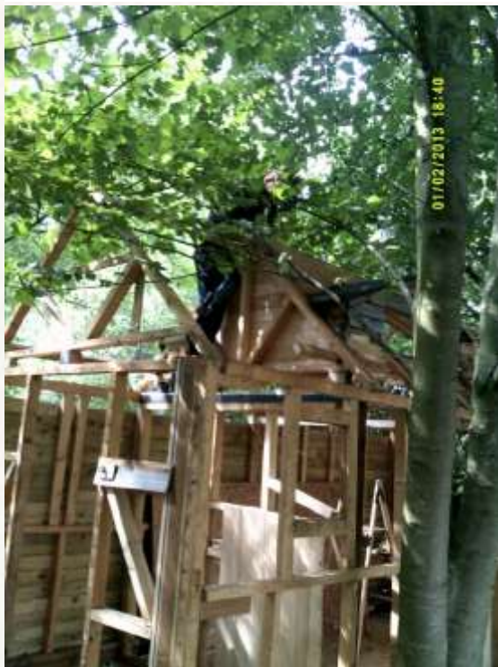
Figure 14. Roof framework nearly complete
