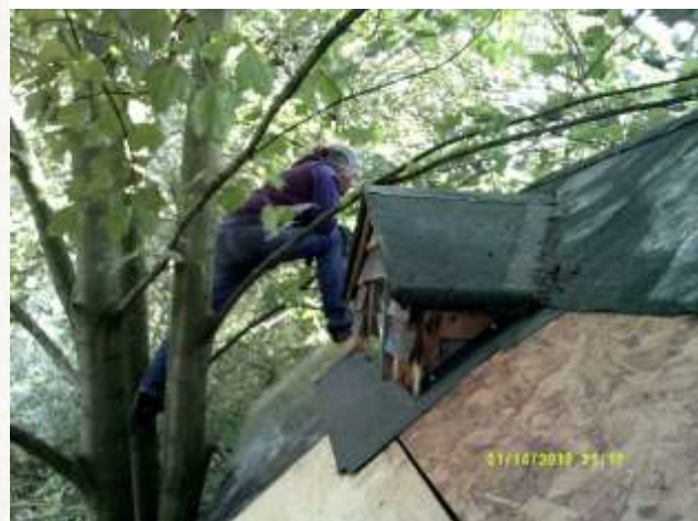
Figure 17. Roofing felt goes on
