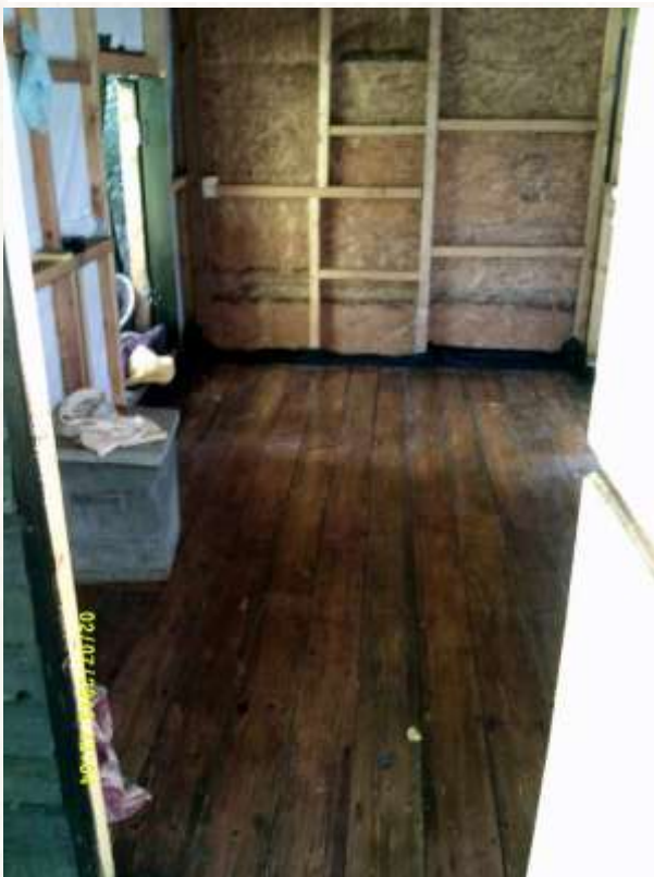
Figure 18. Floorboards laid
