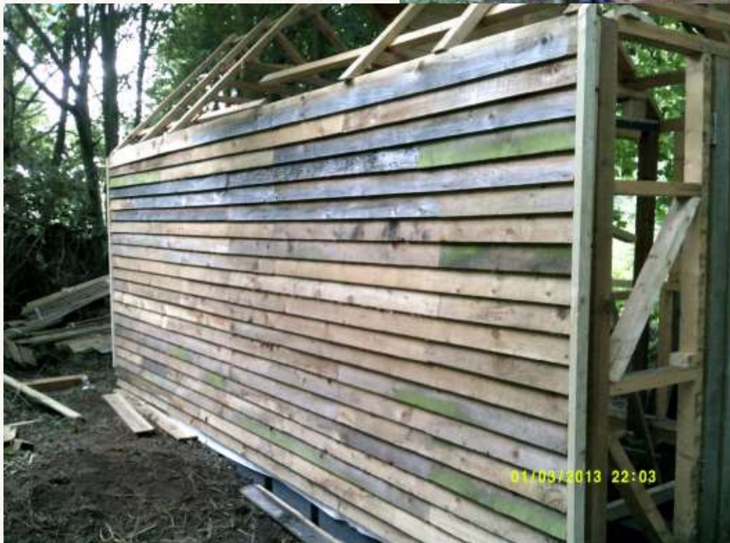
Figure 13. Cladding on back wall
