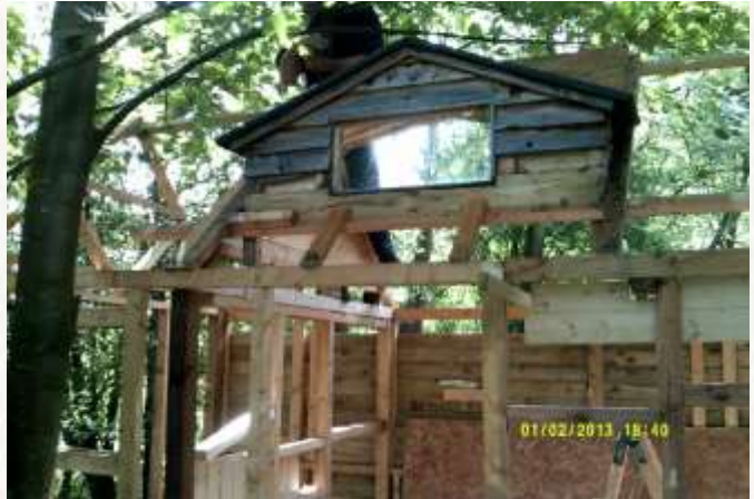
Figure 14. Roof framework nearly complete
